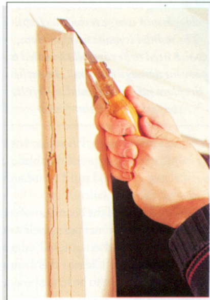
FIG. 1 SLICING NAILS
