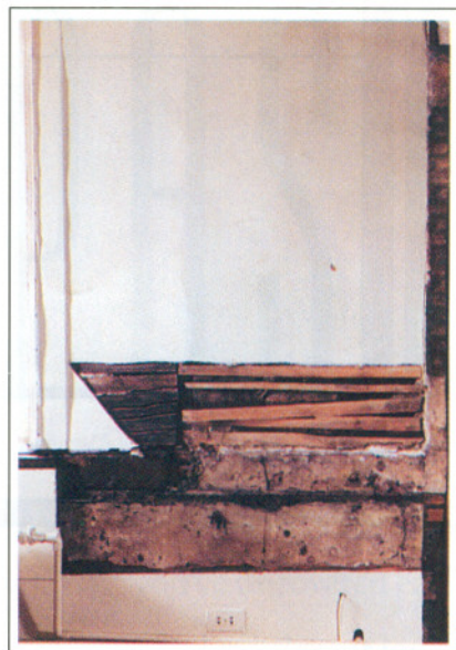
FIG. 3 EXCAVATING THE PLASTER
